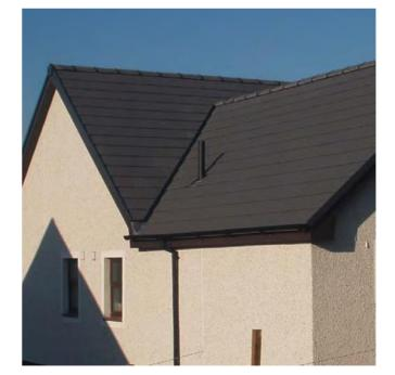
Galloway is a thin leading edge flat interlocking roof tile which has the appearance of a slate when laid broken bonded.
