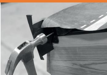
Remove the tile and **Dry Verge Unit** and secure the **Eaves Stop End** with a **Drive Screwnail**.
