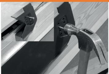
With the back of the **Dry Verge Unit** pressed firmly down, nail through the appropriate hole with a **Drive Screwnail**.
