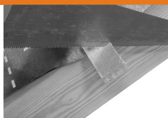
Cut the tiling battens to overhang the verge by 45mm. The underlay should not extend more than 10mm past the verge.
