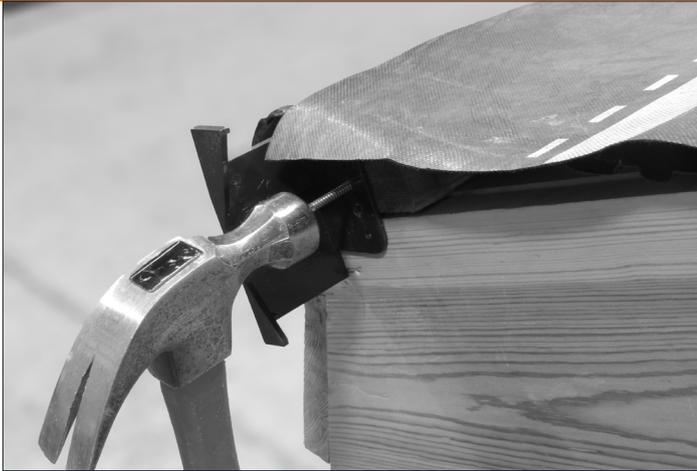
Remove the tile and **Dry Verge Unit** and secure the **Eaves Stop End** with a **Drive Screwnail**.
